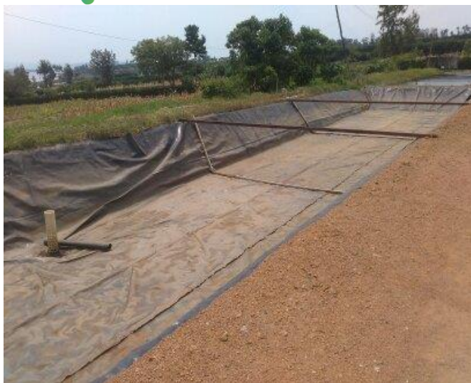
Plate 1: Dug out pond with plastic under lay to reduce water loss during dry season in Rwanda. An adaptation technique in CSA. Source: Field survey 2016
